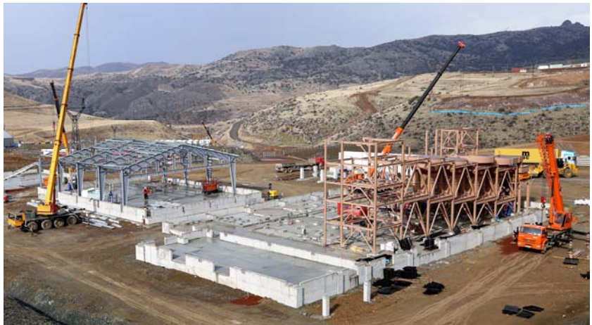
Gold Processing Facilities
